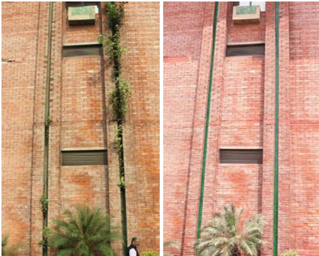
Rainwater Channels (before and after)
